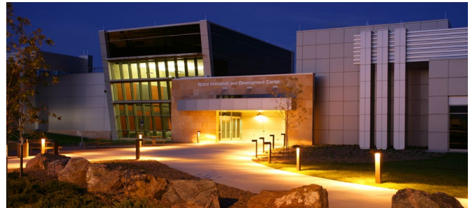
Space Innovation and Development Center, Schriever AFB, CO
